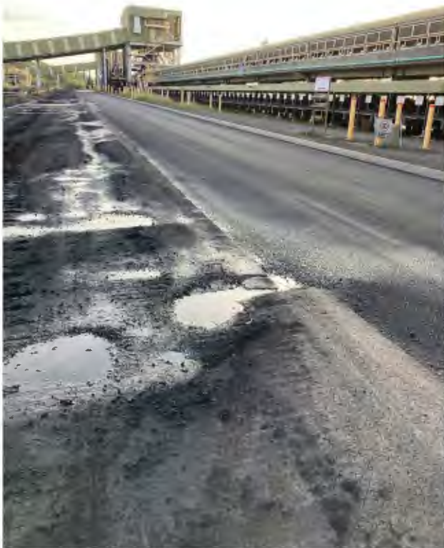
L1 southern lane (before). Typical surface condition
