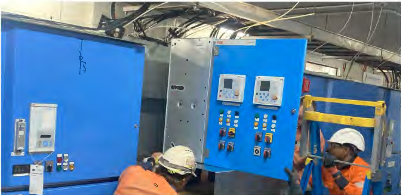
Figure 5 – New remote racking system complete and in operation
