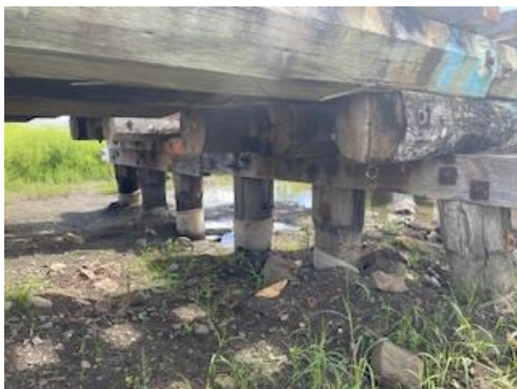
Figure 5-2 WMS timber bridge
