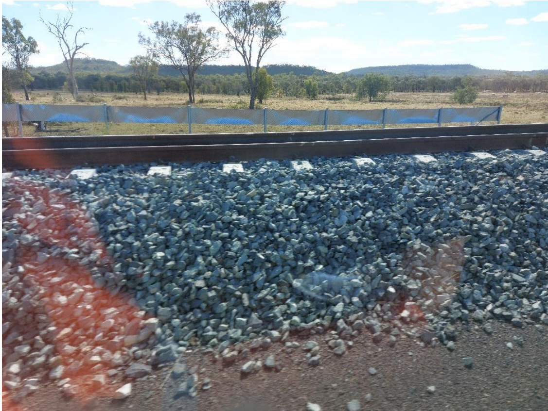
Figure 6-7 Track structure with Koala fence on the northern side
