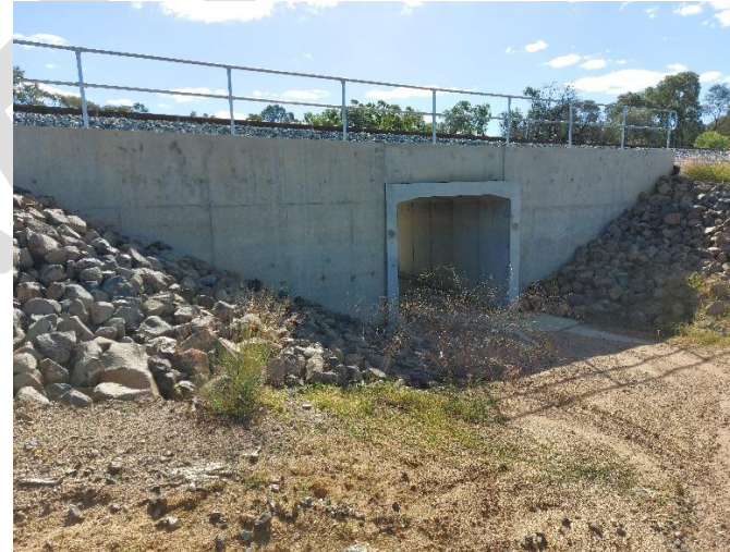
20220726_142324 – Culvert C027_4_up stream
