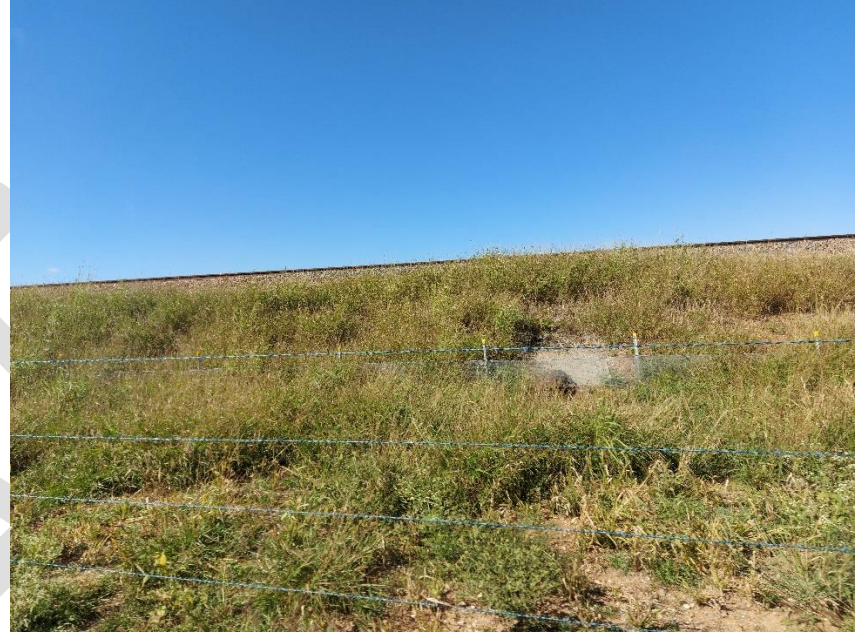
20220726_104827 – Snake fence and culvert
