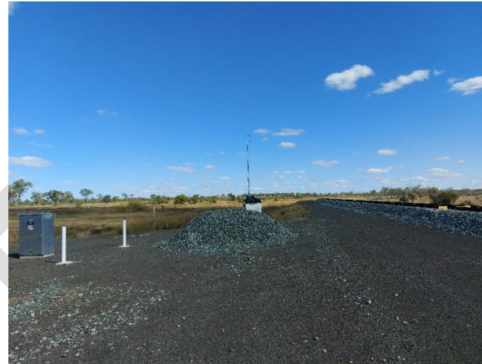
20220726_142425 – Access Road Turn around - Looking West
