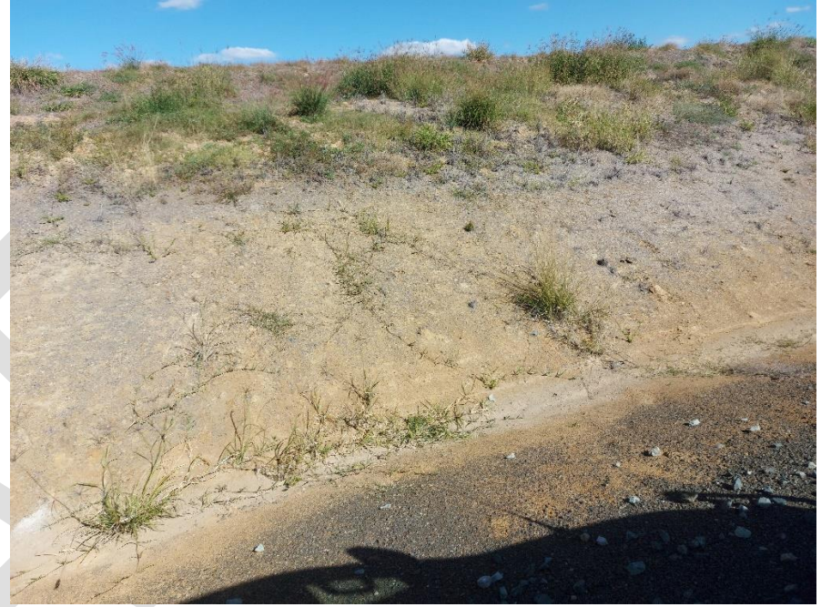
20220726_143655 – Cut and drain near CH 180.700
