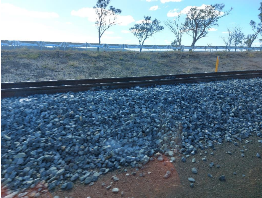
20220726_141057 – Track structure with Koala fence on the Northern side
