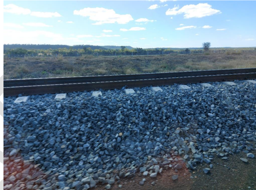
20220726_142324 – Culvert C027_4_up stream
