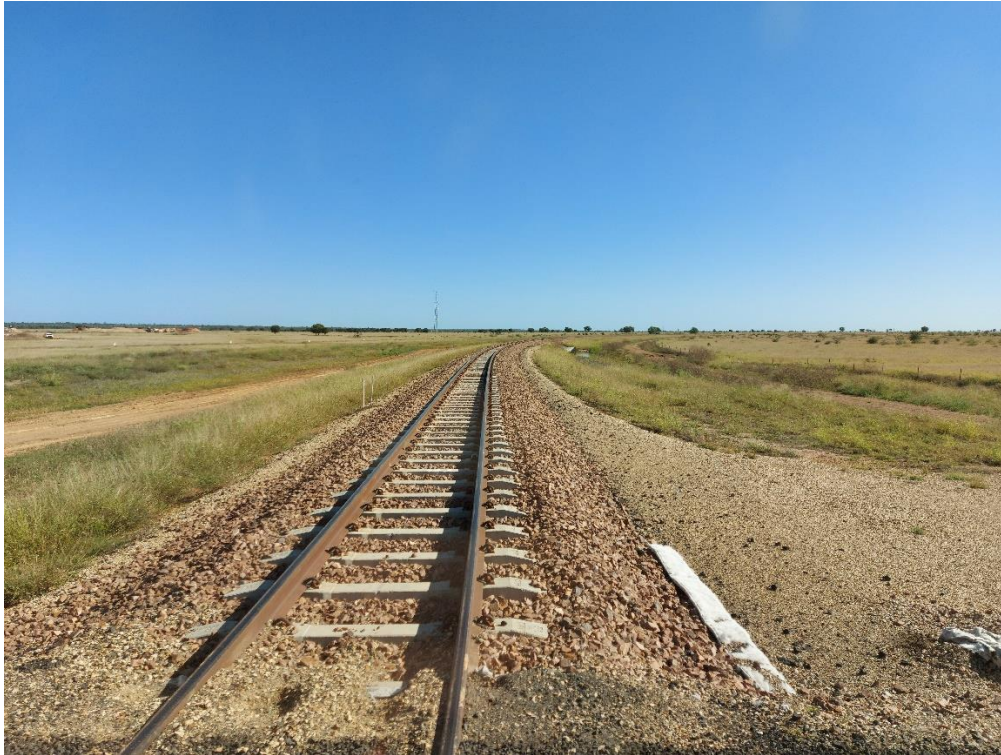
Figure 6-2 60 kg head hardened rail on concrete sleepers
