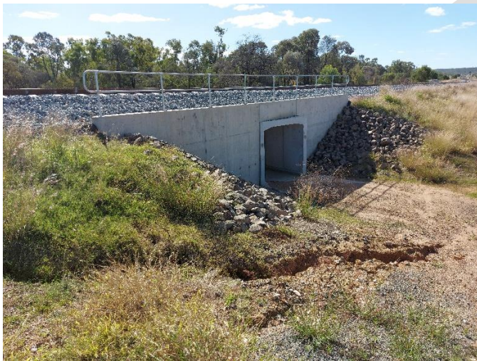
20220726_142250 – Culvert C027_3_up stream
