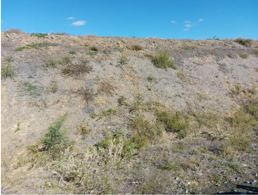
20220726_143655 – Cut and drain near CH 180.700
