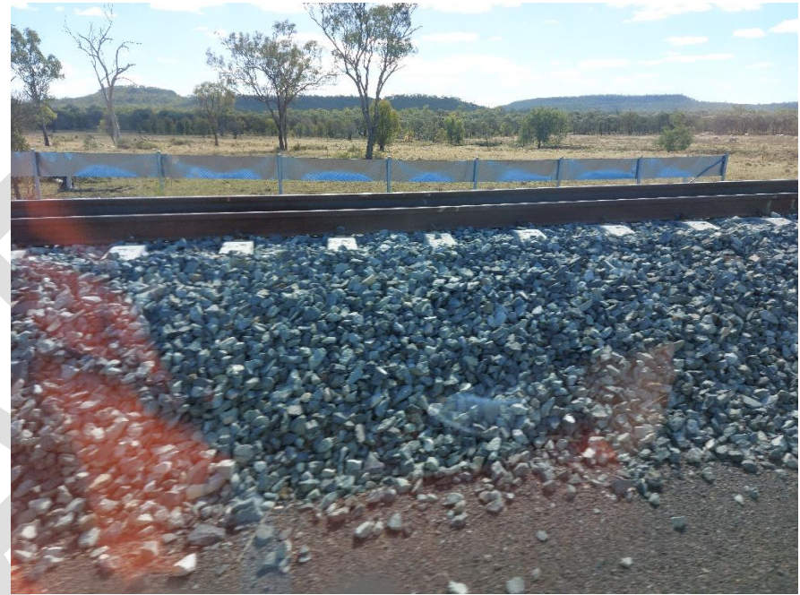
20220726_141142 – Track structure with Koala fence on the Northern side
