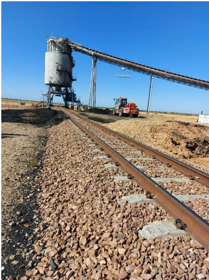
Figure 2-1 Loading facilities and stockpile
