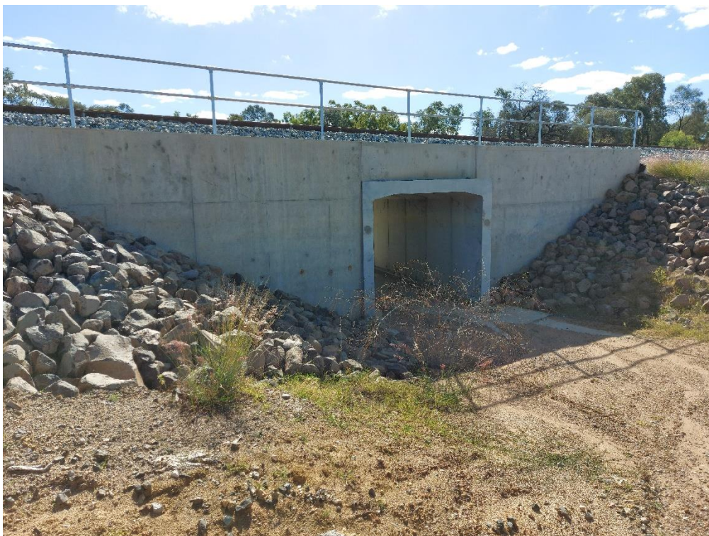
Figure 6-3 Reinforced concrete culvert
