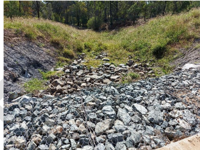
20220726_142415 – Culvert C027_2_down stream
