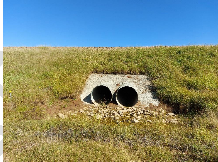
20220726_103554 – Culver C482 at CH 382.906 - 2 x 1.2m CMP
