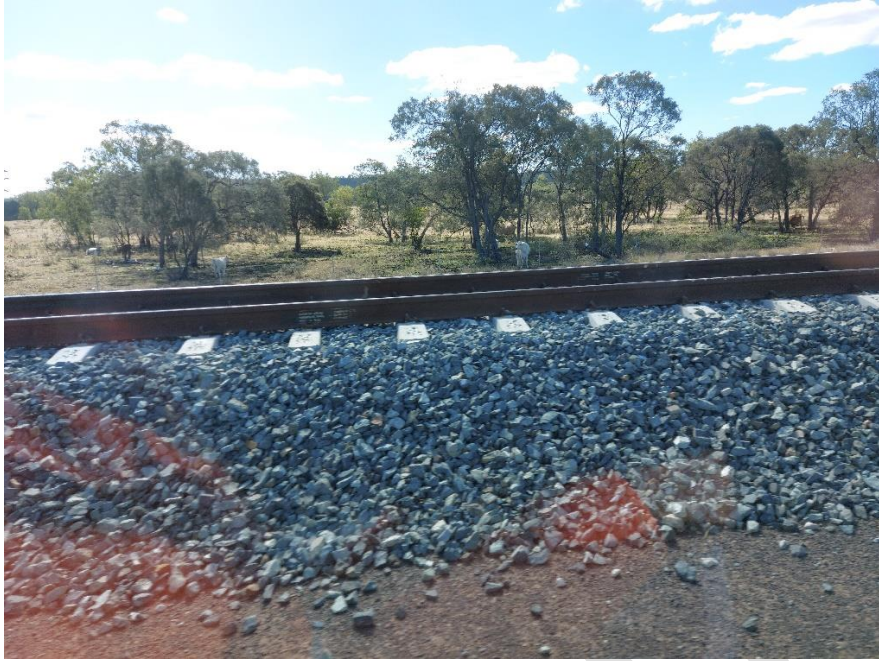
20220726_142250 – Culvert C027_3_up stream
