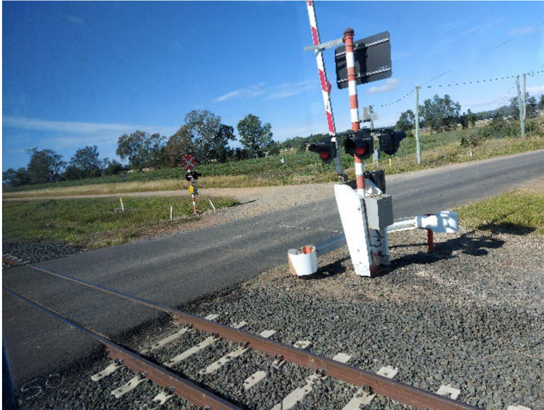
Figure 5-7 Level Crossing Upgrade – Smithfield / Burgess Road (km 98.370)
