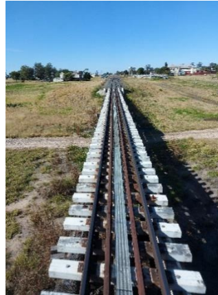
20220621_111203 – Looking East Bridge at km128.100
