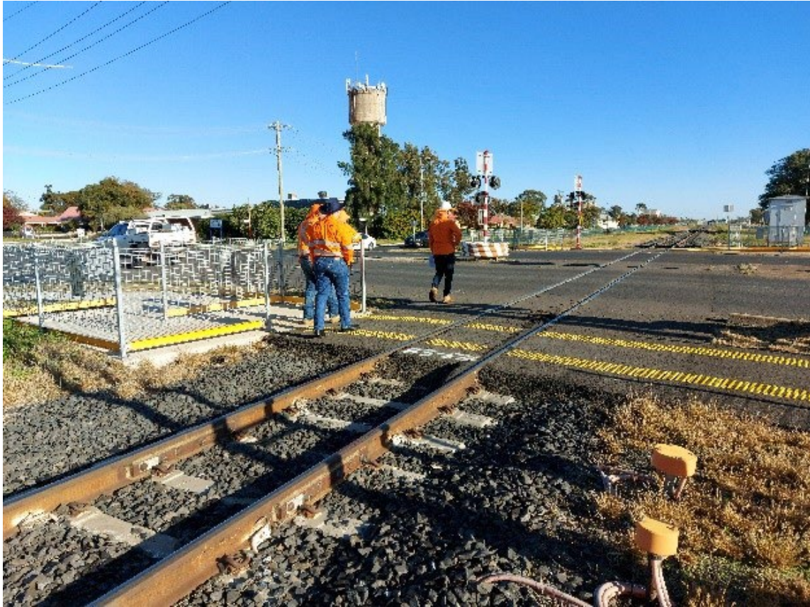
Figure 5-6 Level crossing upgrade at Nicholson Street, Dalby (km. 84.180)
