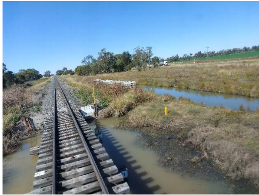
20220621_111324 – Looking East Bridge at km 128.740
