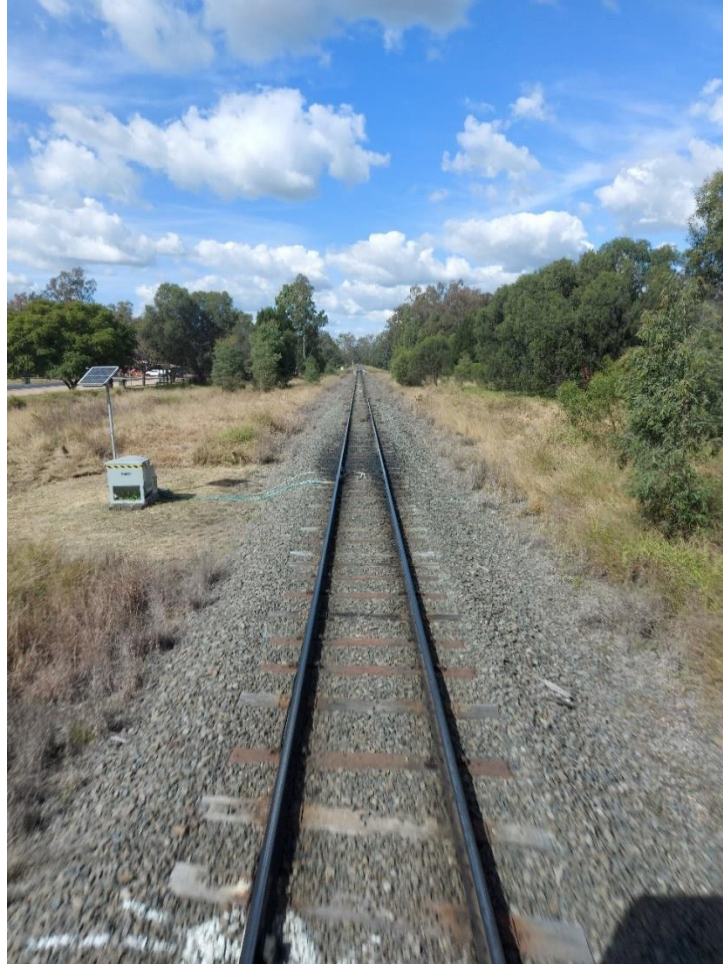
20220621_124703 – Looking East (near km 106.000)
