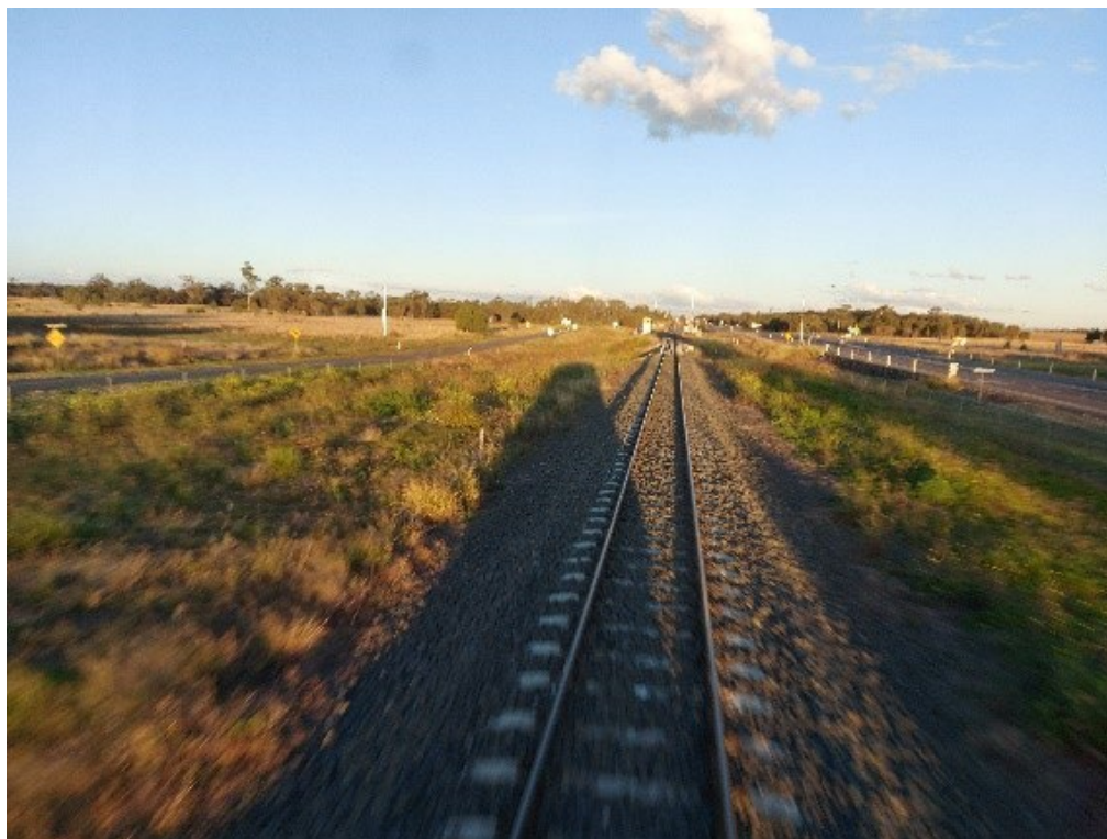
Figure 5-1 Track reconditioning between km 44.570 to Km 48.202 (looking east)
