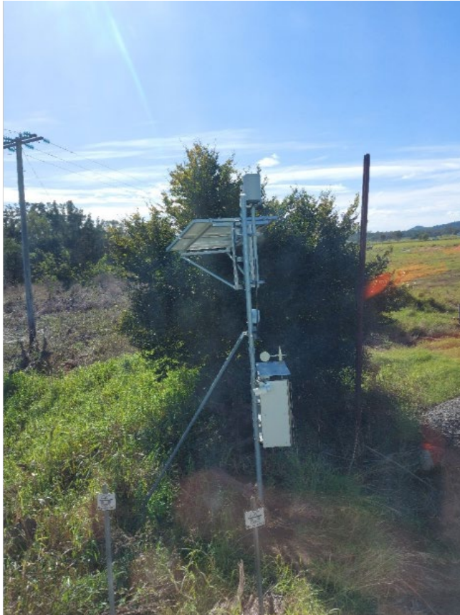
Figure 5-4 WMS Replacement (Regional). 20 June 2022, Looking North.
