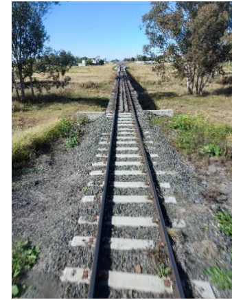
20220621_111215 – Looking East Bridge at km128.100
