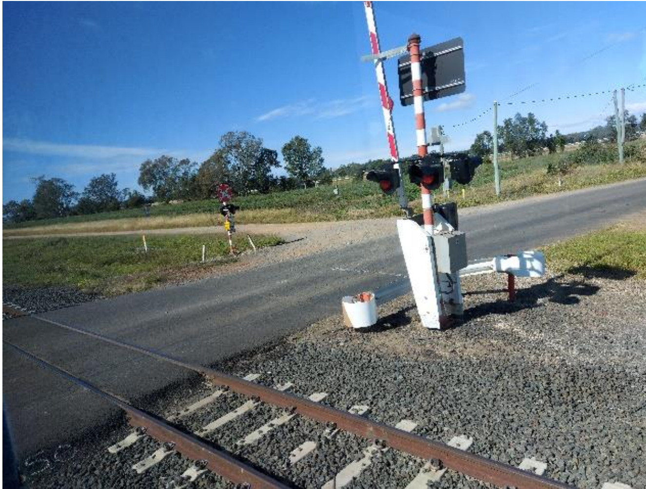
Example to identify/read photograph by Date and time taken - 20220622 – Looking West
