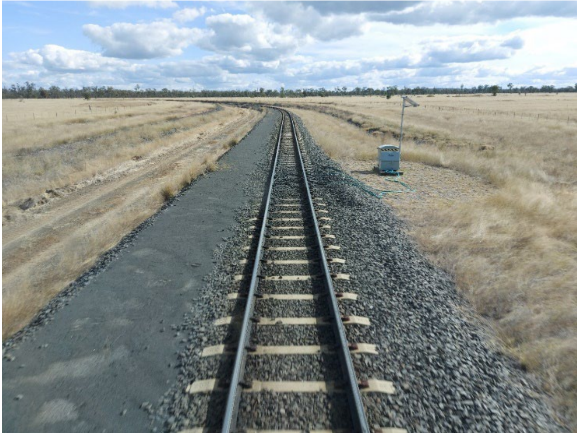
Figure 5-3 Greasers Replacement Upgrades 21 June 2022, Looking East
