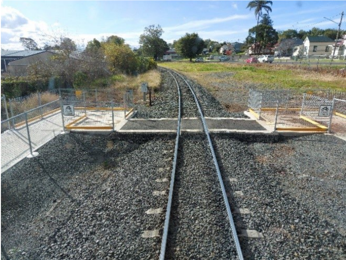
Figure 5-5 Level Crossing Upgrades West Moreton. 20 June 2022, Looking East
