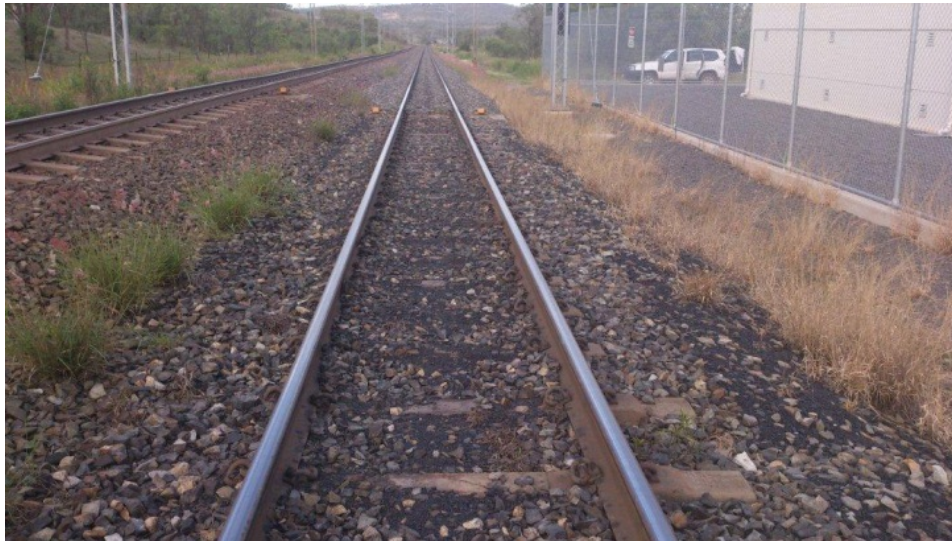
Figure 3: Ballast contaminated with coal spillage
