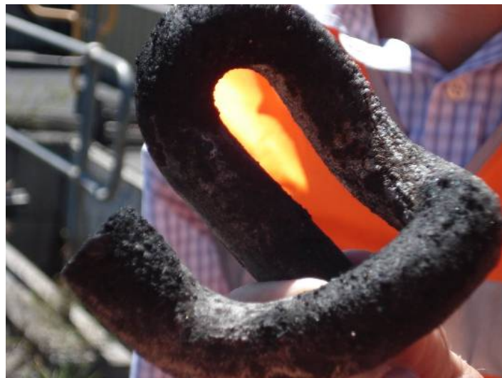
Figure 3 Coal corrodes clips
