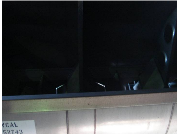
Figure 8 Light can be seen filtering from the bottom of the wagon confirming significant gaps in the doors on completion of the unloading process
