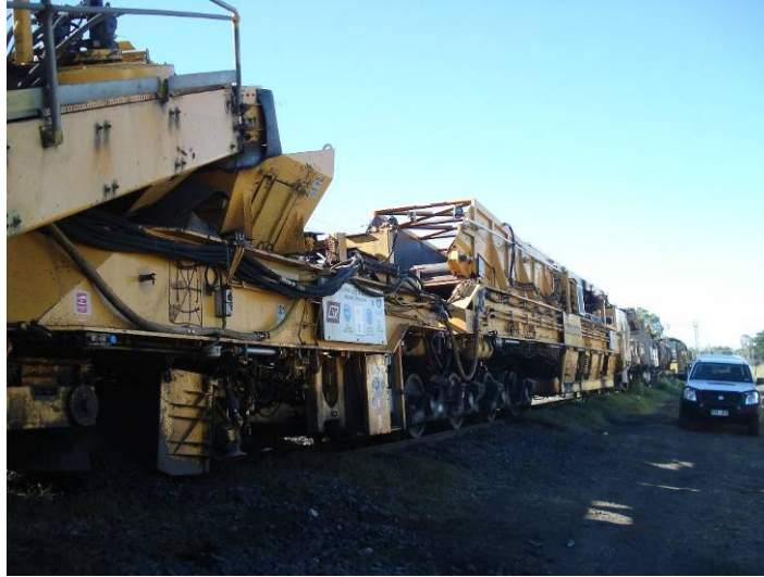
Figure 12 Hauling six ballast wagons; the total length of the machine is 1500m
