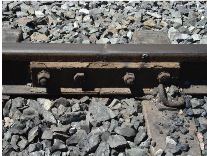
Figure 2 Coal corrodes fishplates
