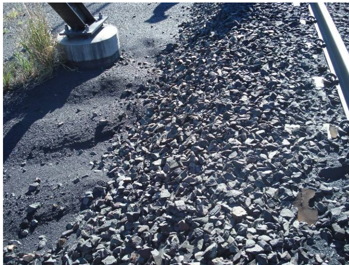
Figure 5 Coal dust contamination - Cess
