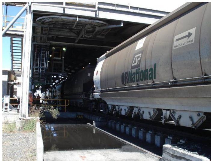
Figure 10 Slab track facilitates cleaning of spillage after unloading processes
