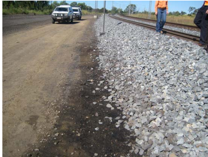
Figure 10 In contrast, ballast from newly ballast cleaned site
