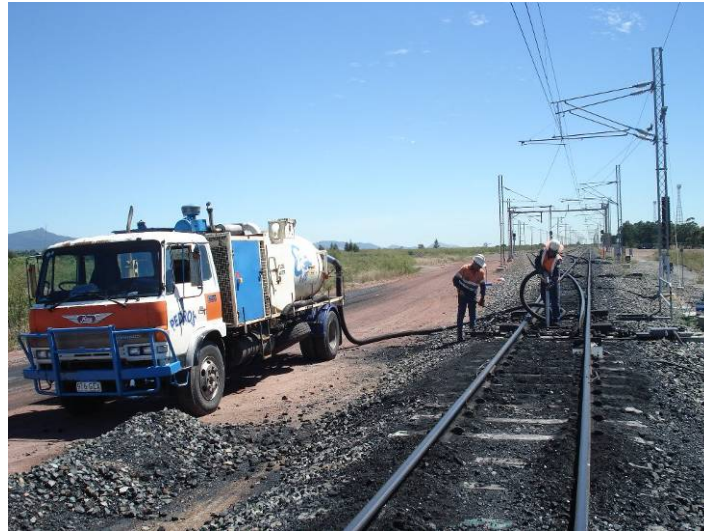
Figure 15 Vacuuming of turnouts
