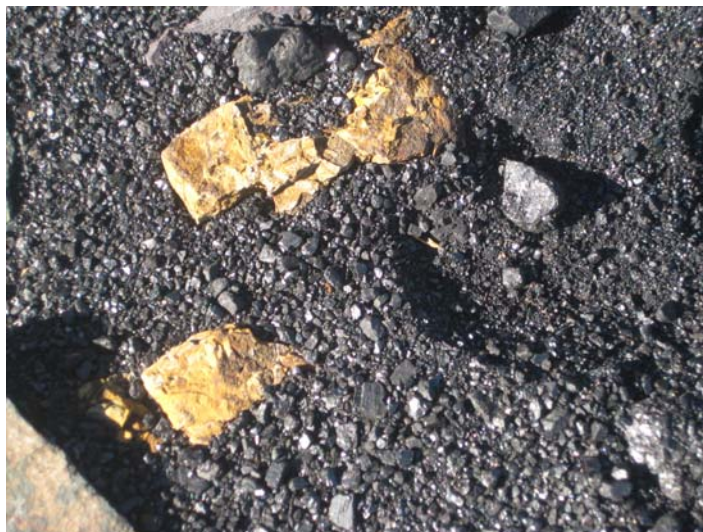
Figure 8 Coal contamination, little remains of the ballast (this location was not near unloading or loading facilities)
