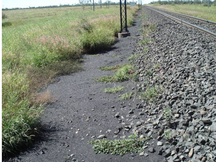
Figure 4 Coal dust contamination of track between mine and port, as can be seen this was taken at considerable distance to unloading & loading facilities
