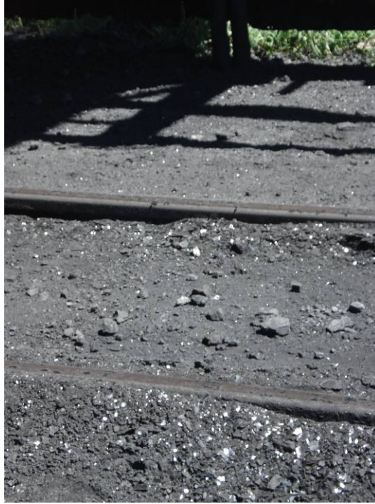
Figure 9 Coal contamination after loading zone
