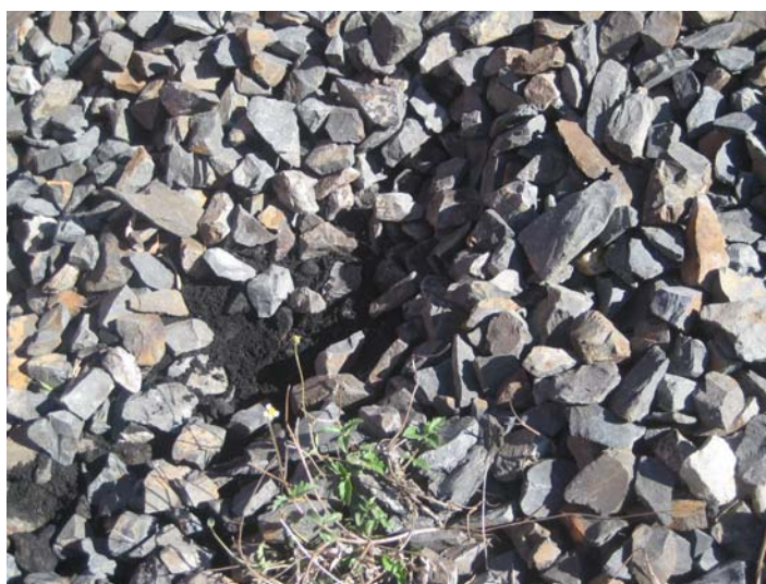
Figure 9 This ballast appears healthier but close examination reveals considerable contamination fairly low beneath surface level
