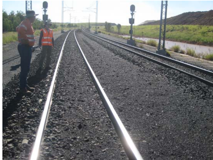
Figure 6 Coal dust contamination approaching accommodation crossing
