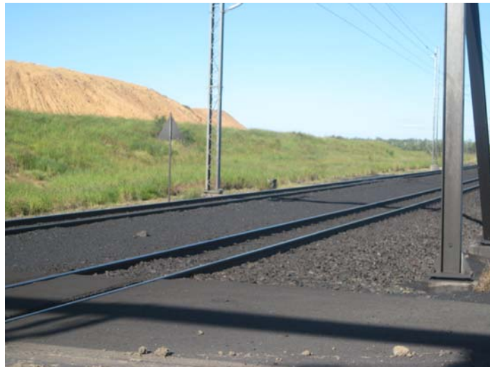
Figure 7 Coal contamination at crossing
