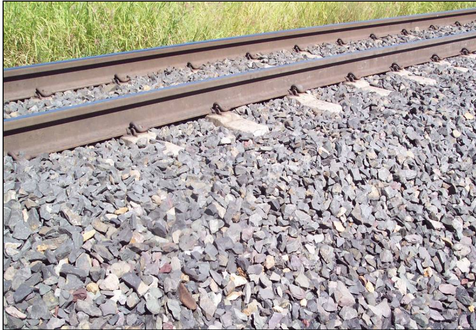
Figure 14 Apparently clean ballast
