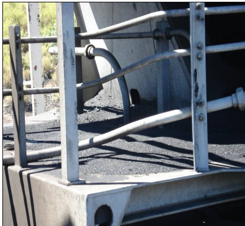
Figure 9 Spillage on wagon surfaces
