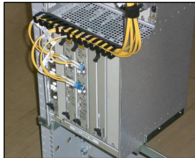
Figure 26 Optical Fibre Multiplex Equipment
