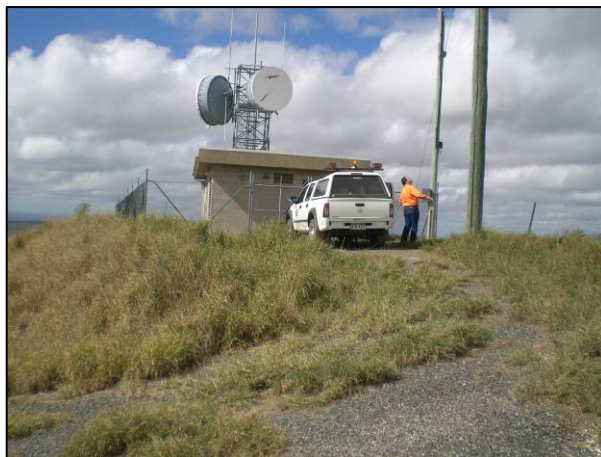
Figure 23 Gogango Microwave Site
