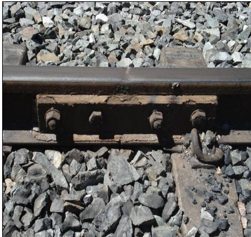
Figure 11 Corrosion to rail furniture
