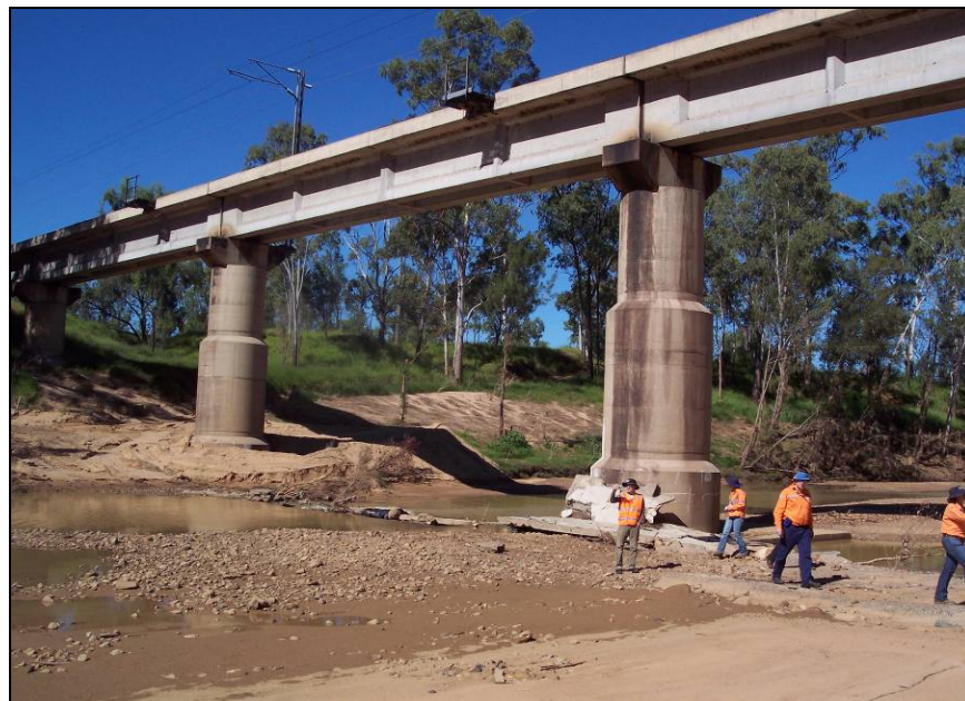
Figure 20 Typical RC bridge. Debris seen consists of roadway washed out in recent flooding
