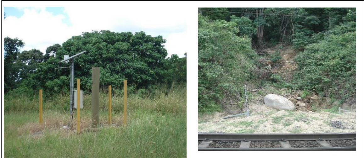
Figure 19 Monitoring rock fall on unstable embankment
