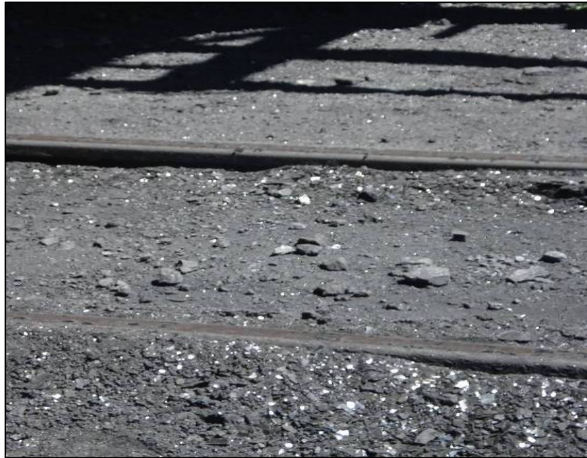
Figure 12 Contamination was severe within loading zones
