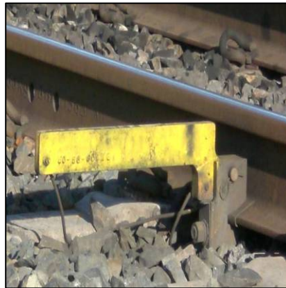
Figure 29 Tryphinia Dragging Equipment Detector
