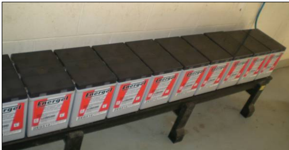
Figure 24 Battery power supply
