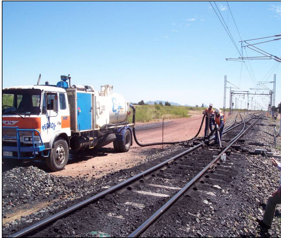
Figure 18 Cleaning of coal contaminates with vacuum system
