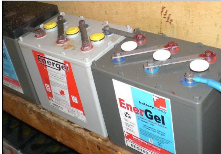
Figure 30 Batteries showing leakage from terminals
