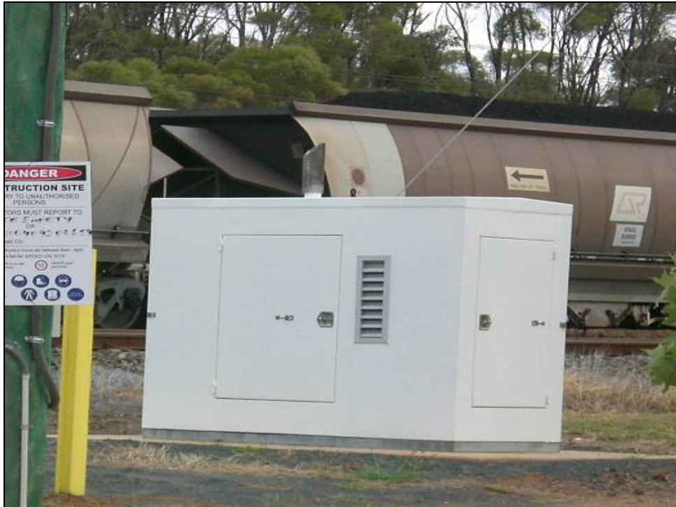
Figure 28 Generator Bluff Station
