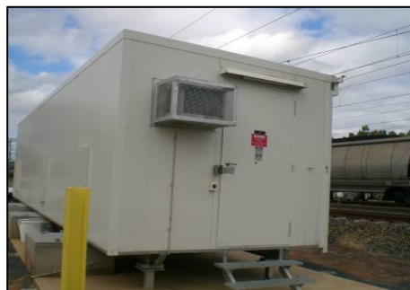
Figure 27 Bluff Station Optical Fibre Site
