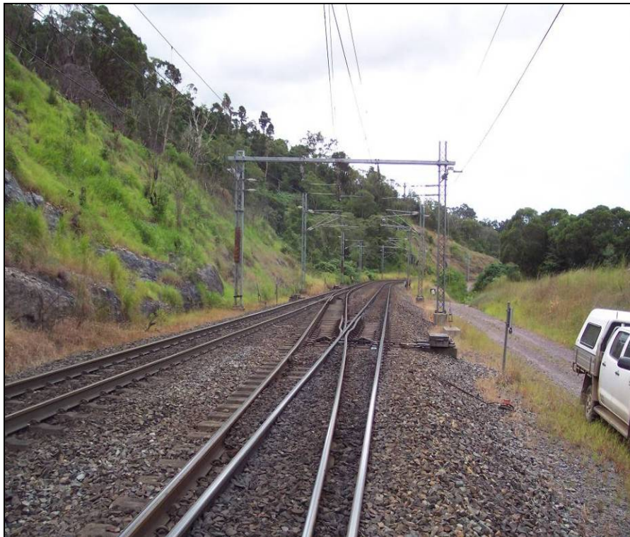
Figure 17 Swing nose turnouts
