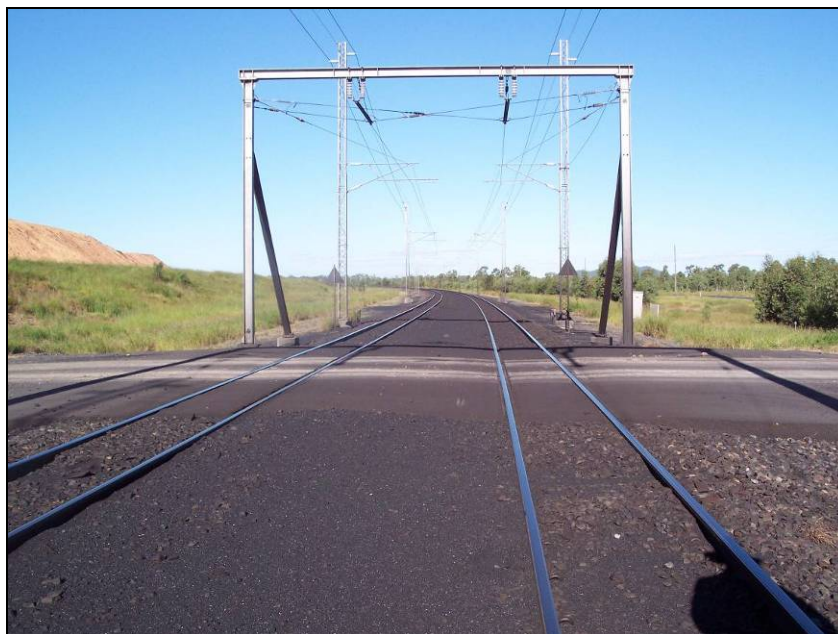
Figure 13 Blackwater main line contamination away from unloading and loading zones
