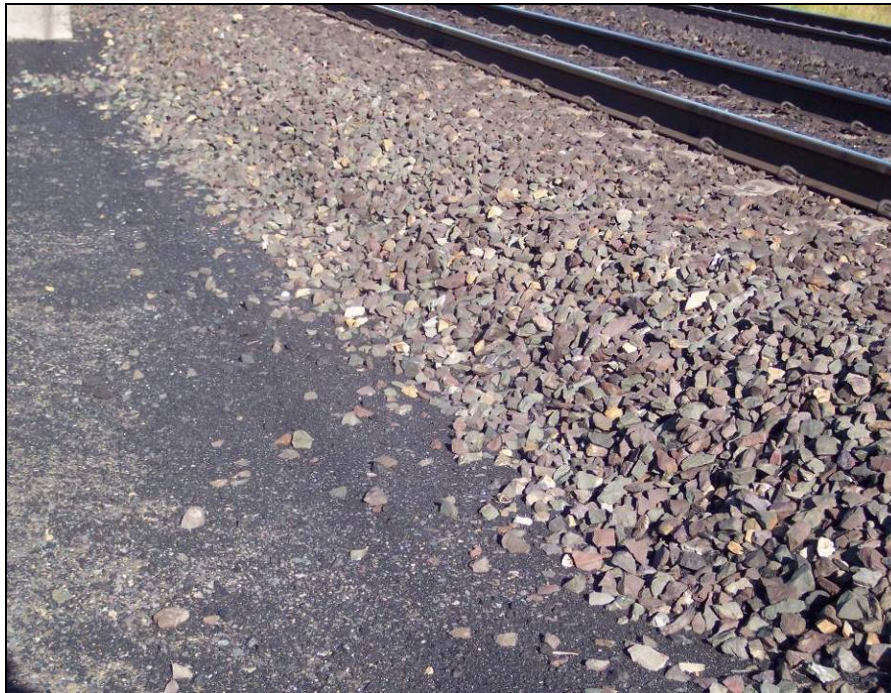
Figure 16 Coal being washed from ballast into cess
