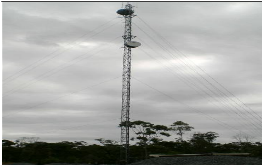
Figure 25 Wallaroo Microwave and Optical Fibre Site
