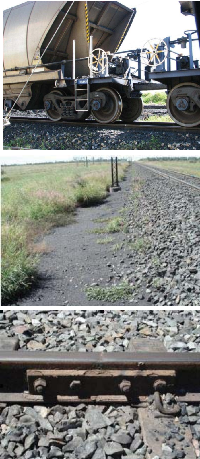
Figure 8: Ballast Fouling on the CQCN
