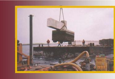
APC is part of a success story that combined major cost savings and environmentally friendly technology. Working in federally-protected manatee waters, APC minimized debris pollution with turbidity curtains surrounding the equipment barge. Water samples taken before, during and after each pile cut revealed minimal disturbance to the fragile environment.
