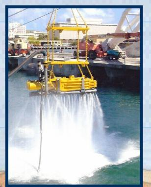
Environmental Concerns? - working in federally protected manatee waters, APC met all environmental standards while cutting and jetting 114 bents with 6-10 piles per bent.
