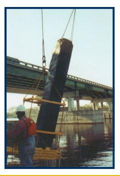
Our pile cutter can safely saw off and gently remove piles located in environmentally protected waterways.
